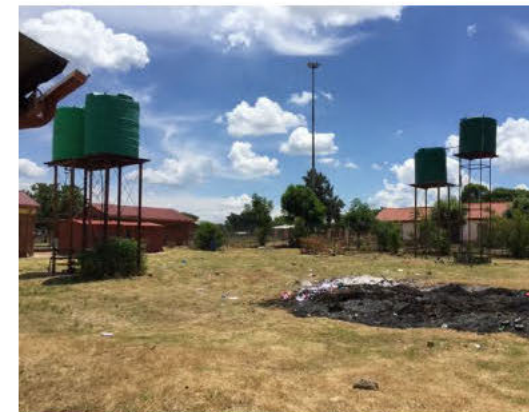
A total of four Jojo tanks were seen on site. All pump water from the municipal water supply.
