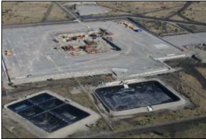
May 2010 - Bulk Earthworks complete
