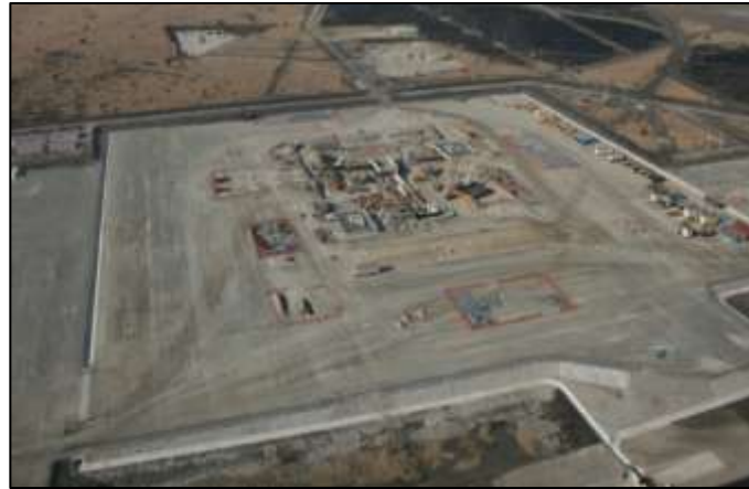
August 2010 - Bulk Civils underway
