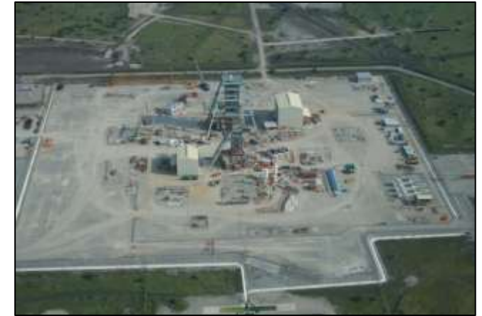
February 2011 - Headgears erected
