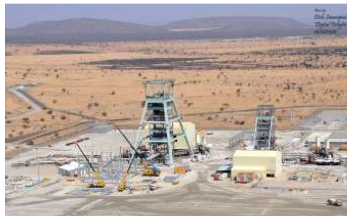
March 2012 - Rock winder civils commenced
