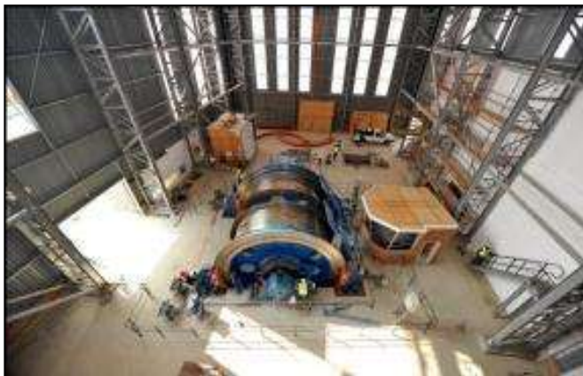
April 2011 - Winders Installed
