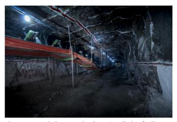
The temporary belt system has been installed to facilitate lateral development rock handling through the Service shaft whilst the Main shaft is being sunk to shaft bottom and equipped.
