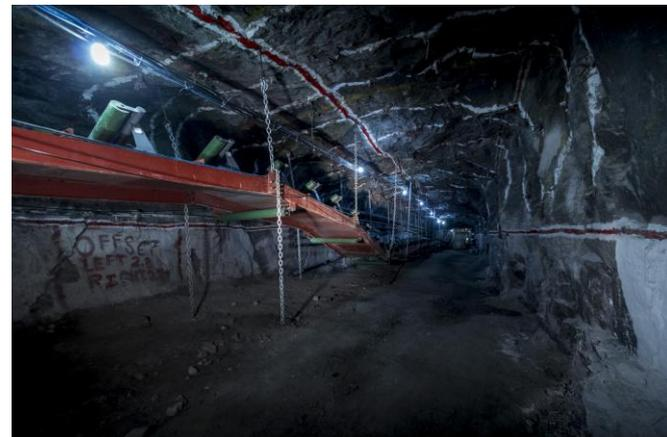
The temporary belt system has been installed to facilitate lateral development rock handling through the Service shaft whilst the Main shaft is being sunk to shaft bottom and equipped.
