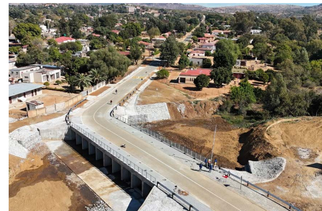
Phokeng after the modern bridge and roadway was constructed, improving community resilience in the face of extreme weather events
