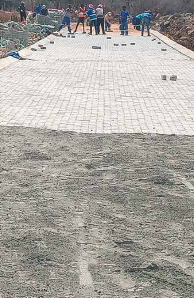
Waste rock from Impala Rustenburg was used in the construction of this road leading to Kutlwanong School for the Deaf
