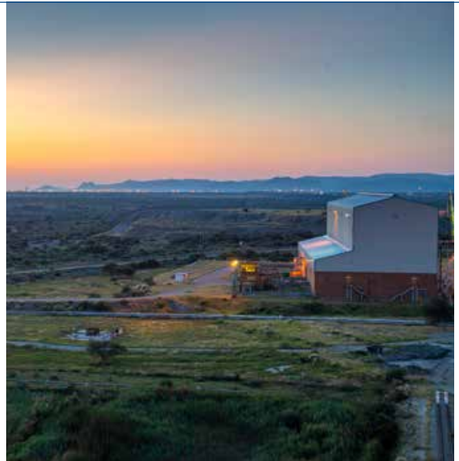
No 14 Shaft winder house, Impala Rustenburg
