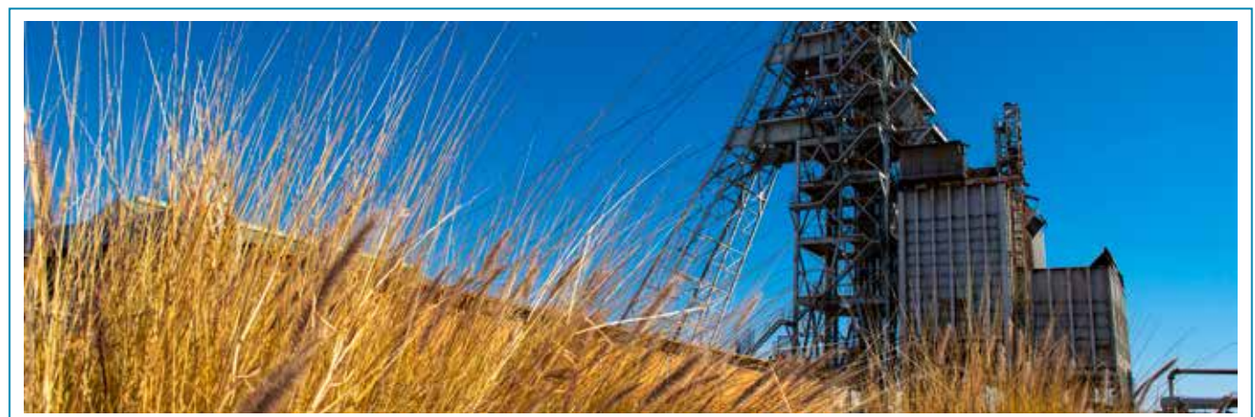
■ No 10 Shaft headgear ■
